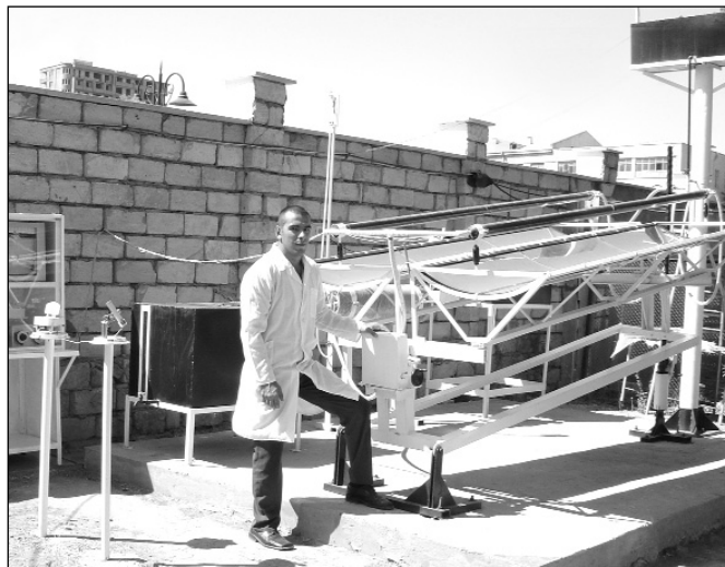
Figure 1. Solar plant with parabolic trough concentrator
