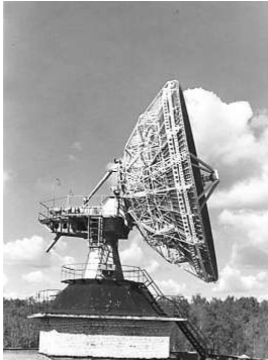
Fig. 3. Full-circle antenna THA-57, 12 meters in diameter. It will be placed on Mashuk mountain
