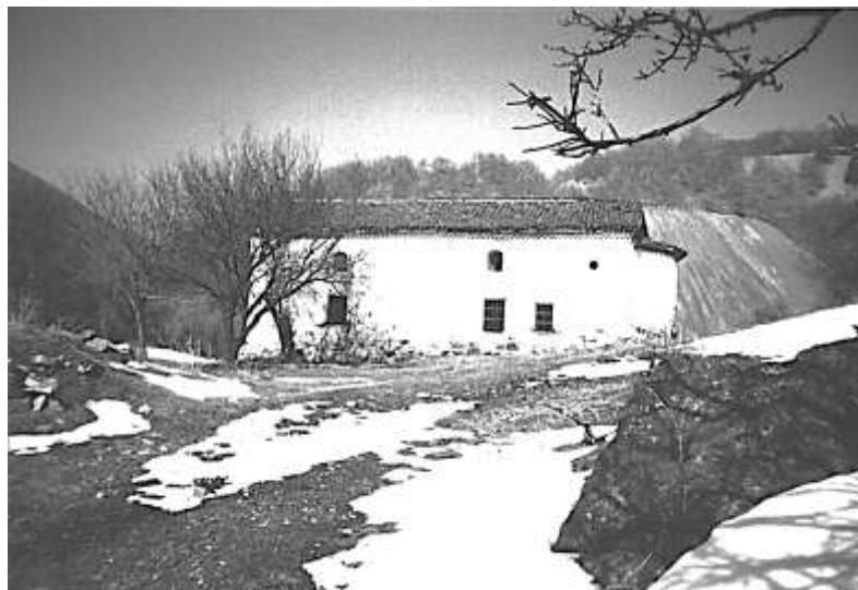
Fig. 8. The Seslavtsi monastery (W Bulgaria) that was damaged by a number of man-made earthquakes, and seemingly by natural quakes as well
