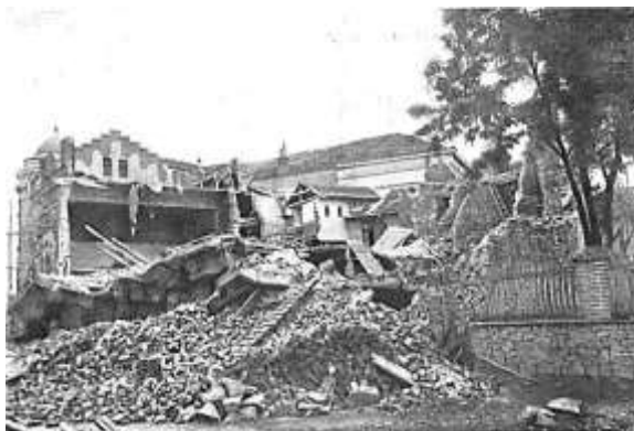
Fig. 6. Destruction of representative buildings in Plovdiv City as a result of 1928 Popovitsa earthquake (M 7.0) [1]
